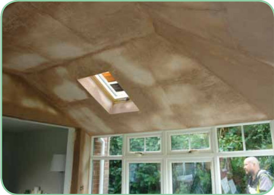
Step 7. Standard thickness foil backed plasterboard fitted onto battens, before taping and skimming.
