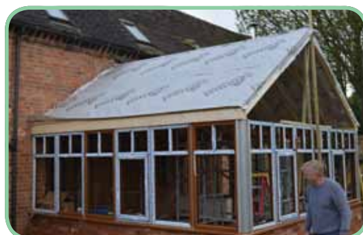
Step 4. Waterproof air permeable felt membrane attached - roof already waterproof within hours.
