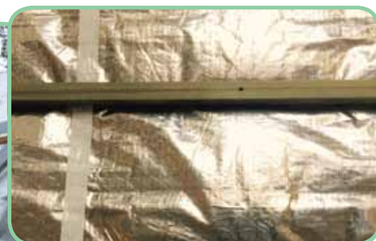
Step 6. Internal vapour barrier attached and secured in place with 50mm x 50mm horizontal battens.
