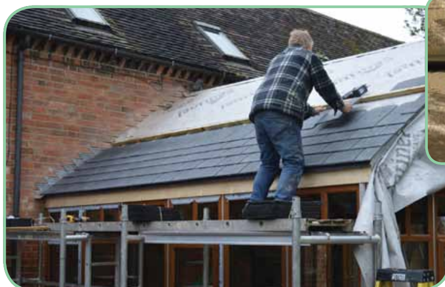
Step 5. Eaves protection fitted and tiling can begin ahead of fascia board and gutter fixing.
