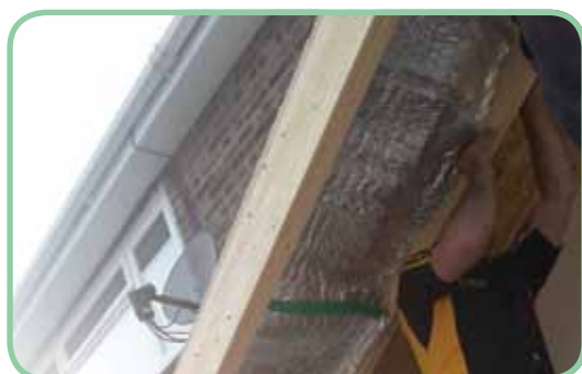
Step 3. Individual pods including pre-cut and fitted insulation located, glued and bolted into position.
