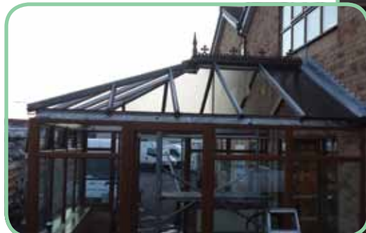
Step 2. Glulam eaves beam goes on.
