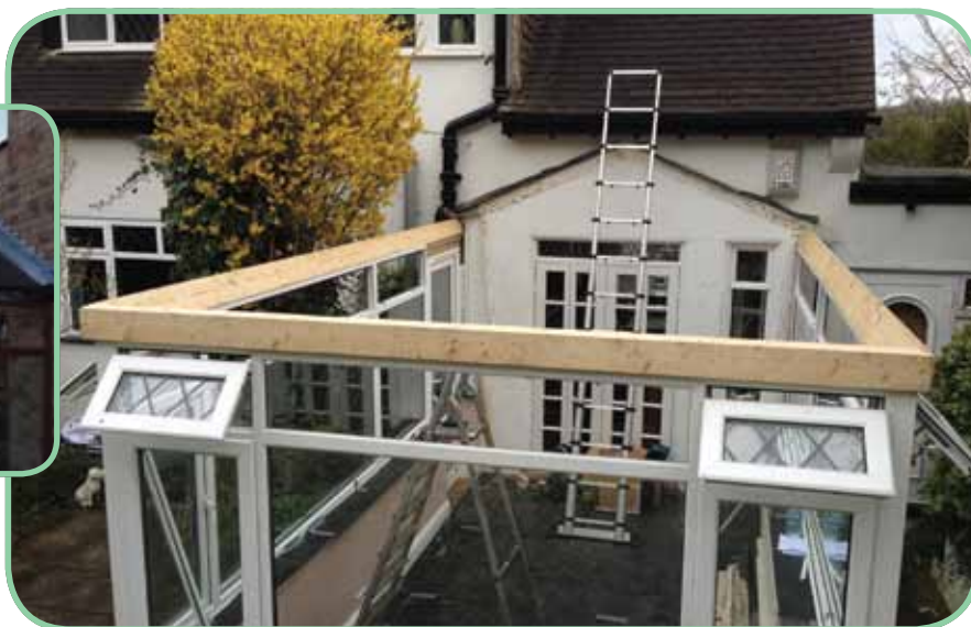
Step 2. Glulam eaves beam goes on.
